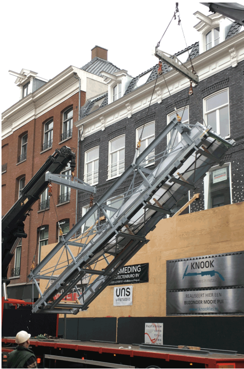
The frame arrives horizontal on site and is rotated to be mounted vertically in the facade.
